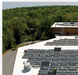
Completed Phase I of campus solar installation project
