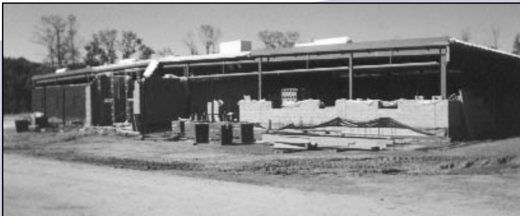
New field house nearing completion
