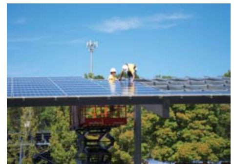
Workers install solar panels over the athletic field parking lot.
